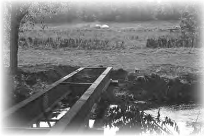
A bridge under construction across Wilson's Creek.
